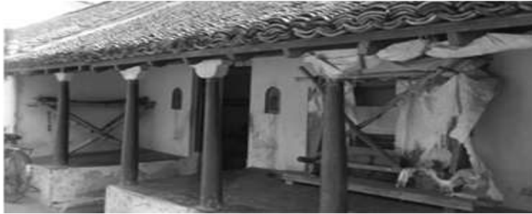
Entrance door with Thinnai on both sides
